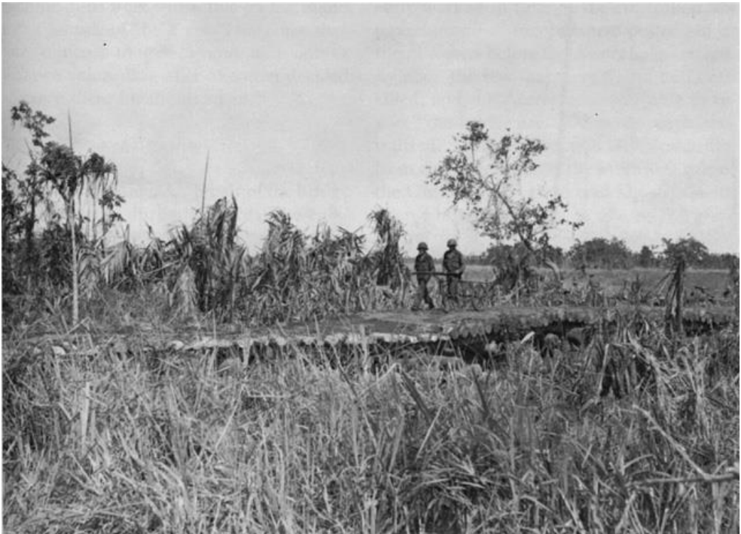
The Simemi Creek Bridge. This is clearly not much of a bridge and is meant for only foot traffic. It is also an easy point for Japanese fire to concentrate on and US infantry would be limited to that bridge as it is surrounded by jungle. 11
