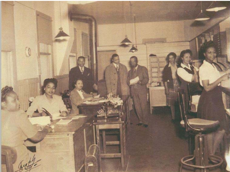
Figure 2. A view of the offices of the auxiliary Boilermakers A-36 Union, a segregated union hall for African American shipyard workers in Richmond, California. Photograph by E. F. Joseph, RORI 686, National Park Service.
